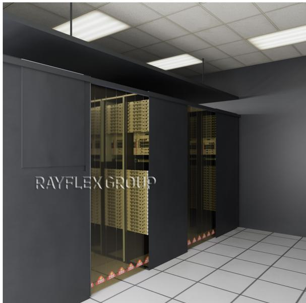
Our Data Centre PVC strip curtains are designed to create a containment seal around your rack space without introducing static and to effectively separate your hot and cold air aisles.
